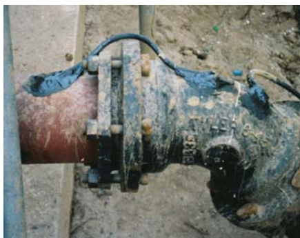
Ductile Iron Pipe w/Mechanical Joints
