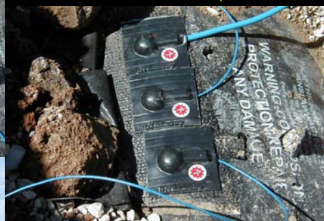
Finished Connections Ready to Backfill
