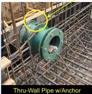
No isolation of pipe-rebar
