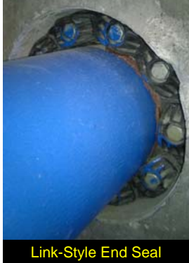
Thru-Wall Pipe w/Anchor
