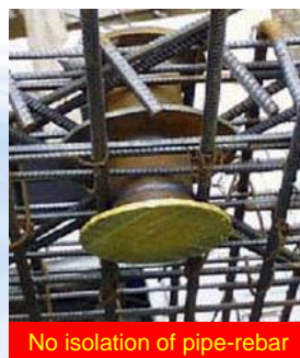
Thru-Wall Pipe w/Anchor
