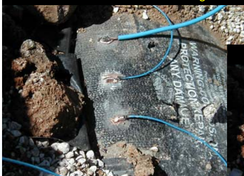
Raw Connections before Coating
