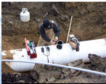
Steel Pipe w/Rubber Gasketed Joints
